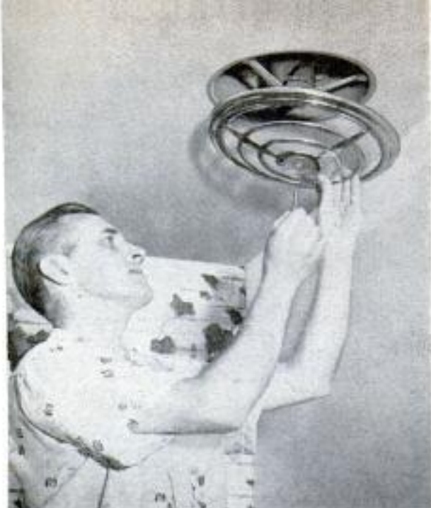
Periodic cleaning of this 10-in. ceiling fan requires unscrewing single thumb bolt to remove grille, unplugging fan and lifting out latter as shown below
